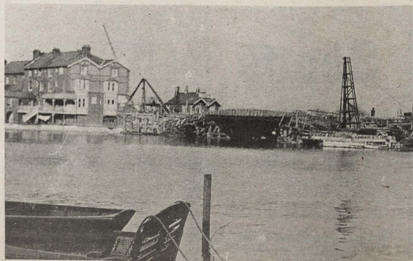
■ The building of the present Caversham Bridge in progress 1924-1926.
