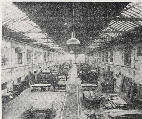
The Machine Mill at Elliotts.
