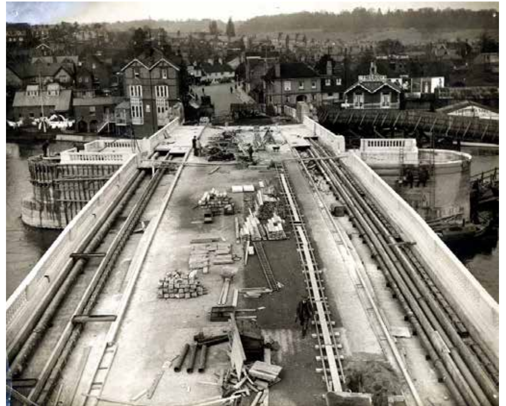
Work is nearing completion with ducts laid for utilities, granite parapets are being installed, to the right is the temporary footbridge and beneath, the new link to Pipers Island can be seen. Courtesy of Reading Libraries
