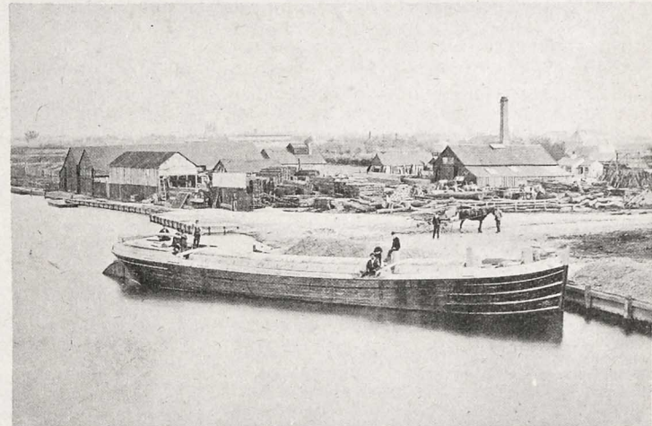
■ One of the giant barges built by R. Talbot and Sons.
