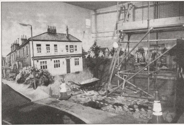
A Building Site
