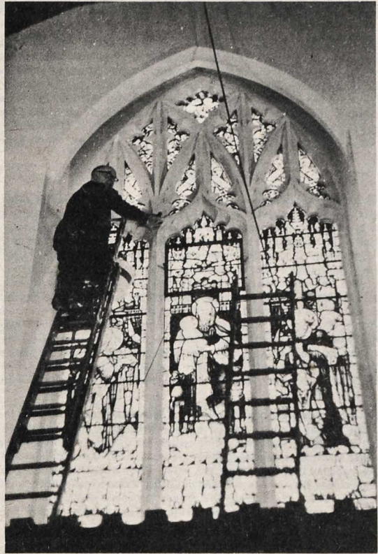
Work in progress at St John's
