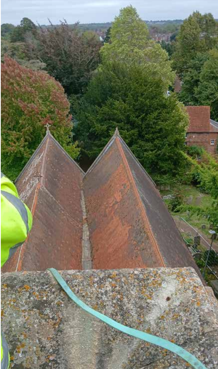
Surveying St Peter's roof from the tower
