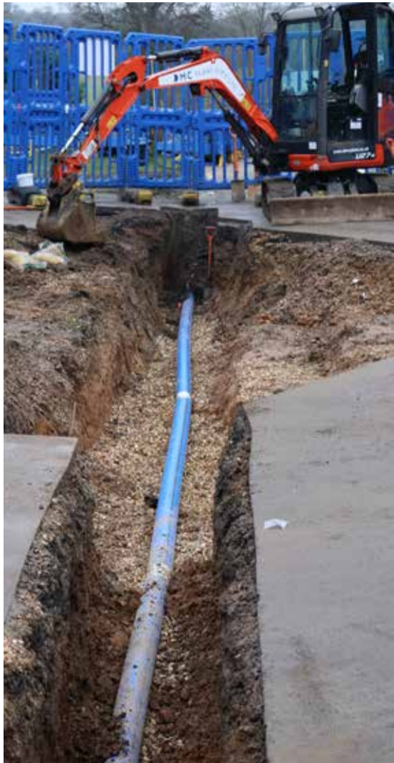
The new water main
