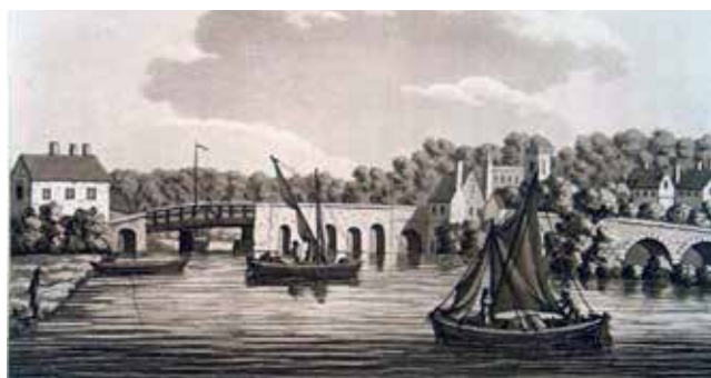
Old Caversham Bridge
