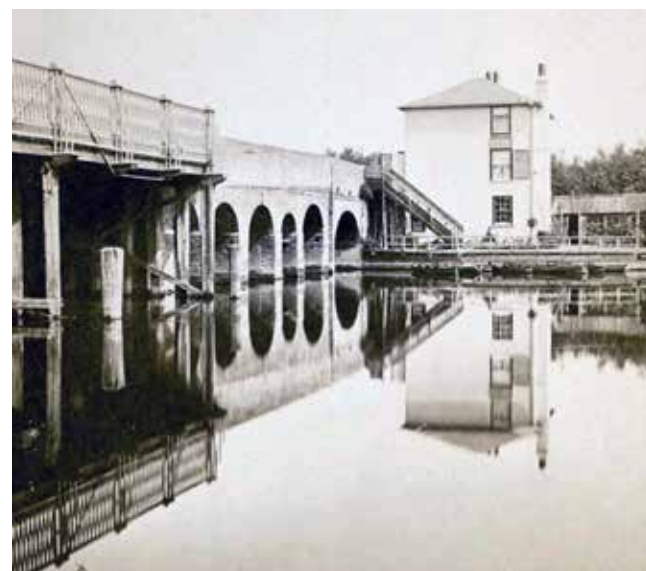
Old Caversham Bridge
