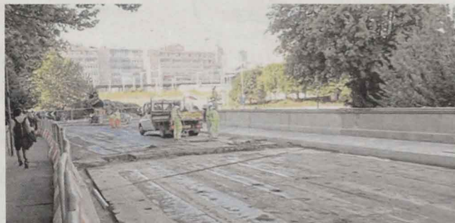
Reading bridge seen while it was closed and under repair
