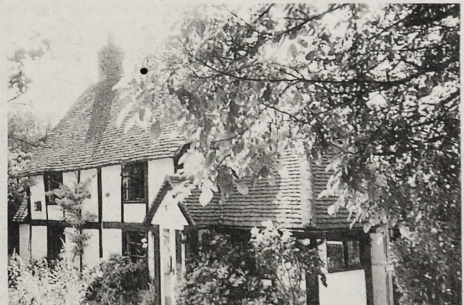
Old Cottage, Lower Henley Road
