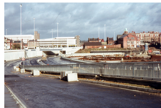
Inner Distribution Road during construction
