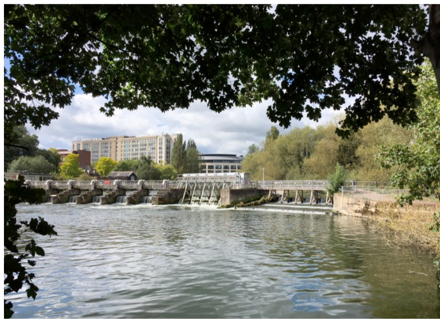
Photo: Reading Hydro The turbine will be placed under the path and to side of the weir
