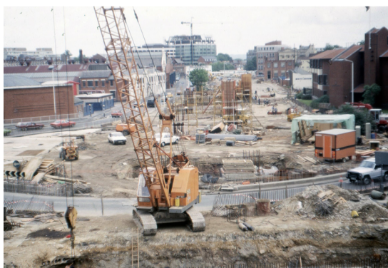
Construction of the Mill Lane fly-over
