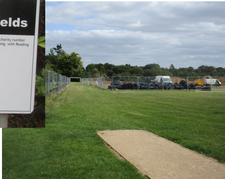
The contractors take over the Fields
