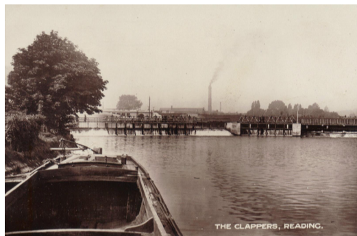
'The Clappers weir looking west'
